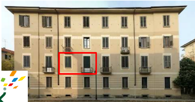
Flat retrofitting Italy- Turin
