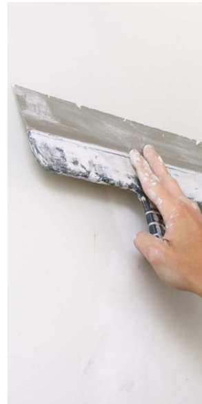
Thermal Coating Finishing
