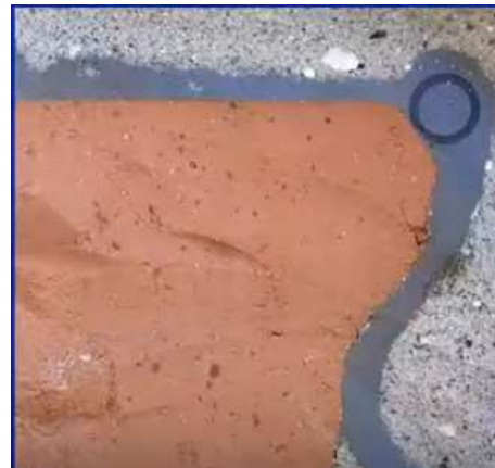
Use of flexible polymer to repair a crack between masonry and concrete (Flex&Robust website)
