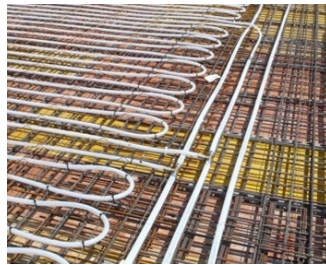
Thermally active slabs
