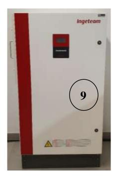
LFP battery DC-DC Converter / Charger (30 kW. 627 Vdc - 800 Vdc)
