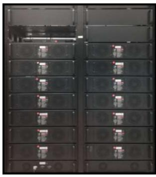
LFP battery DC-AC inverter (30 kW 400 Vac)
