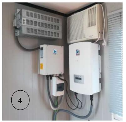
WT DC/DC converter (5 kW. 630 Vac – 800 Vac)
