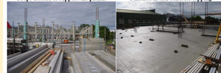
Props erected to support the planks
