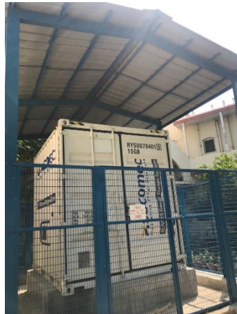
Socomec BESS 200kW/274kWh
