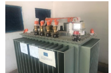
MV/LV Smart transformer with OLTC
