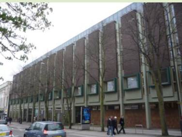
Richard Crossman Building
