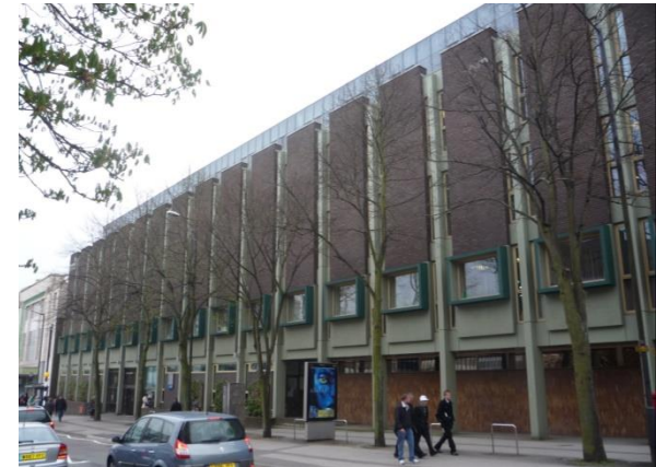
Richard Crossman Building
