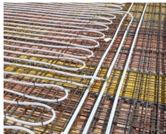
Thermally active slabs
