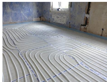
Radiant heating and cooling
