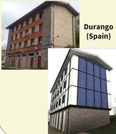
Renovation of real residential buildings
