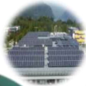
Photovoltaic system 150 kW
