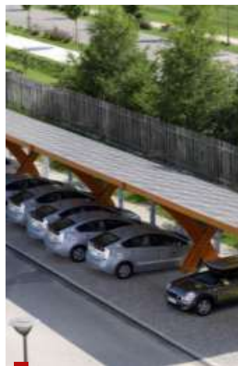
Power electronics Energy management
