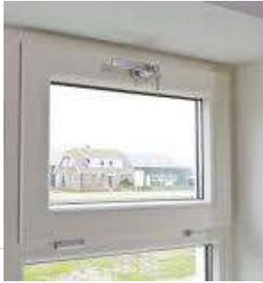
Bedroom windows closed
