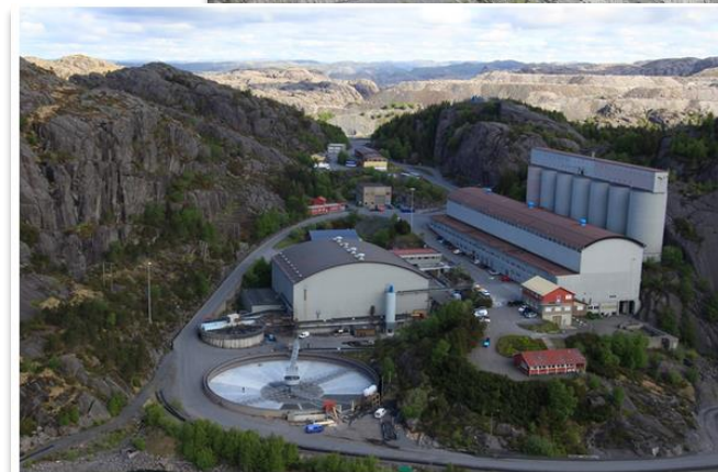
Hommedal Mineral Processing plant
