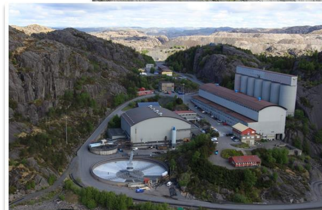
Hommedal Mineral Processing plant
