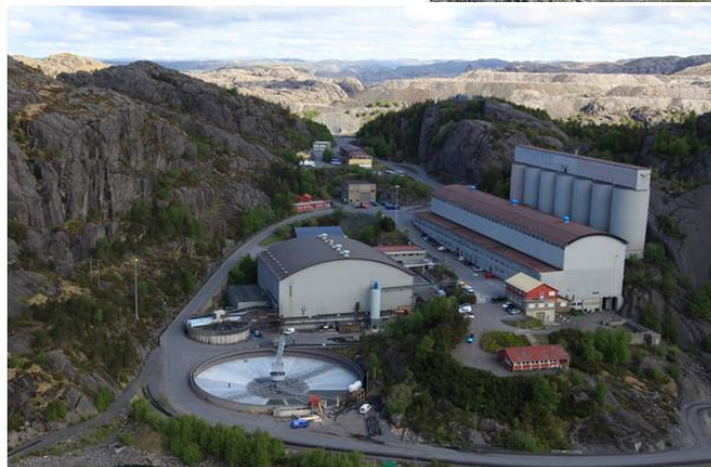
Hommedal Mineral Processing plant
