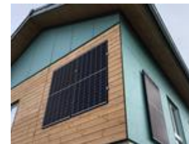
colored PV tiles or façade with tight cladding system
