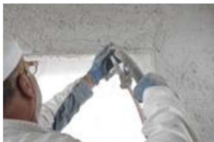
Wood-fibres insulation
