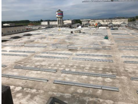
Beams for substructure
