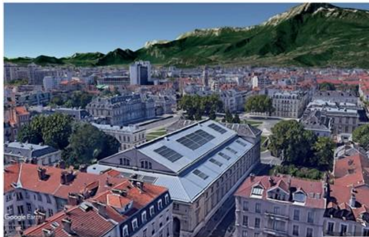
Southwestern view of the building – source Google Earth
