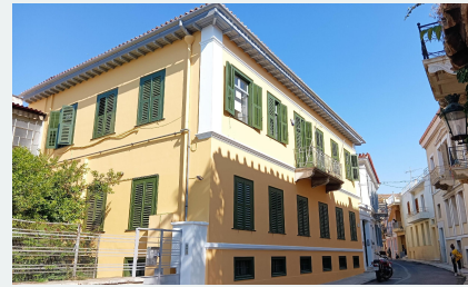
ELLET building in Tripodon Street City of Athens, Greece
