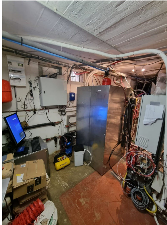
Heat Battery installed in the house basement
