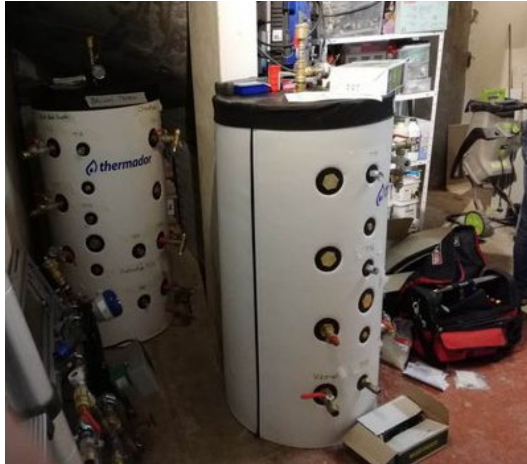
Water tanks used for heat distribution in the house
