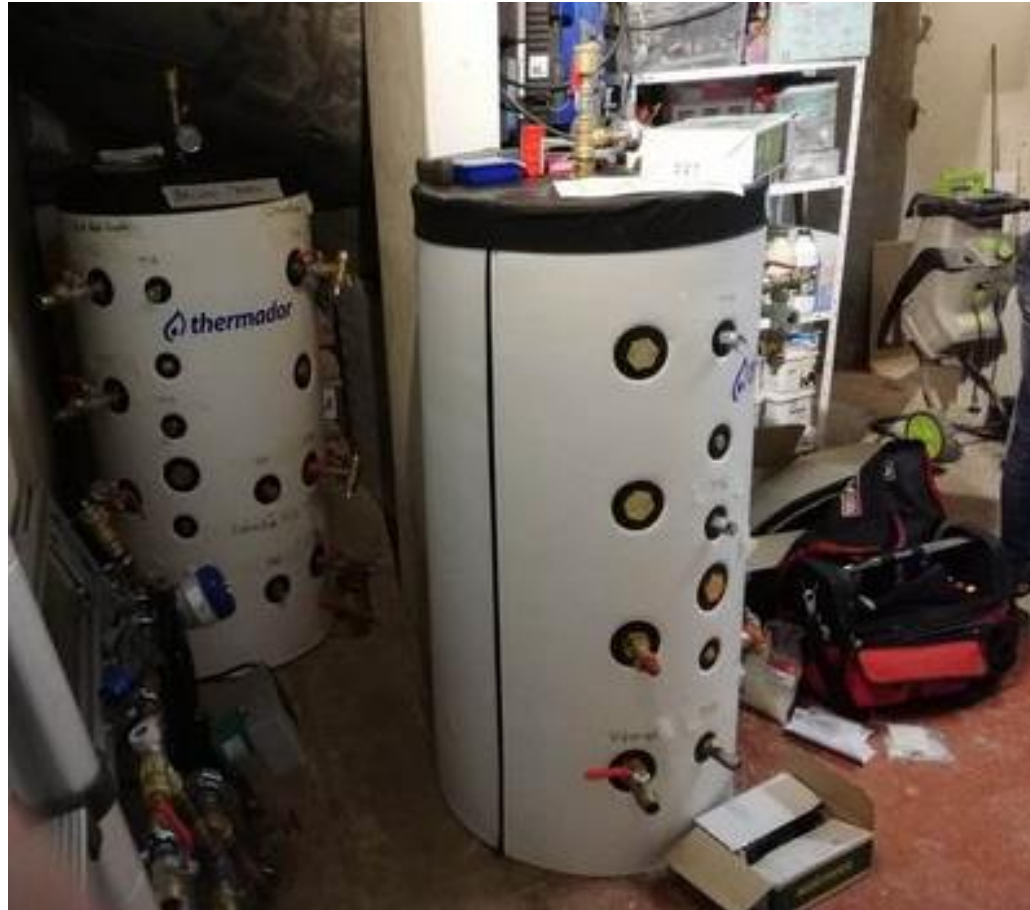
Water tanks used for heat distribution in the house
