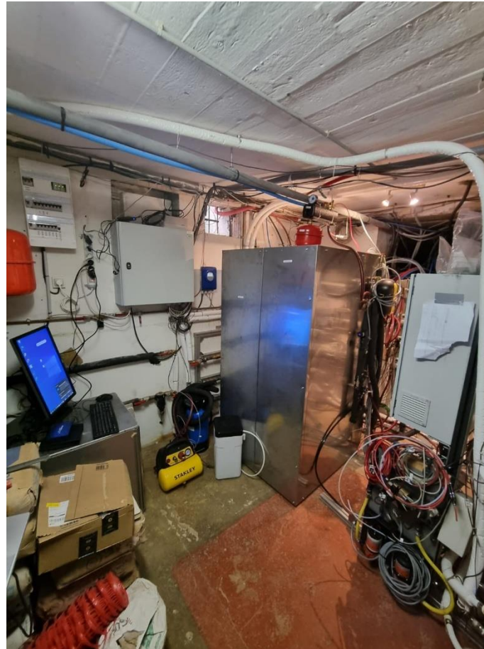
Heat Battery installed in the house basement
