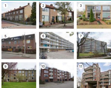
Balcony access buildings – 60s/70s
