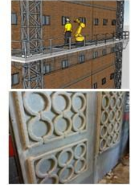
Façade 3D printer Autonomous system for vertical printing onsite
