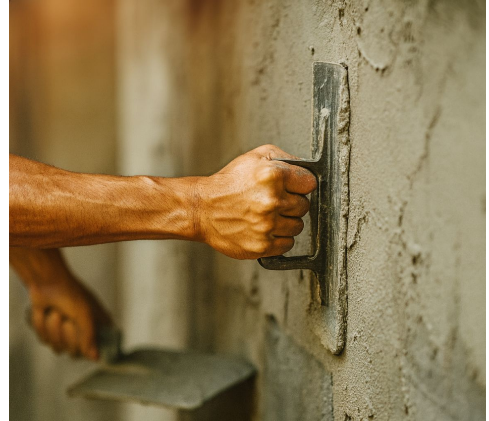
Traditional mortar application execution
