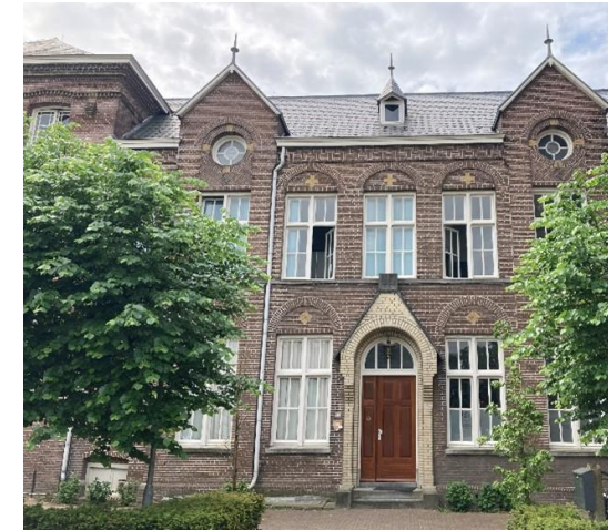
DC#2. Social shelter, The Netherlands
