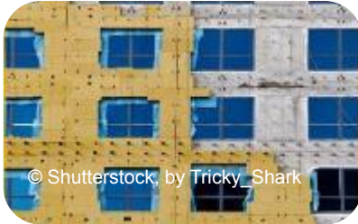
Deep renovation (NZEB, ZEB)
