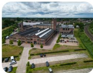
The Netherlands Hazemeijer complex heritage site
